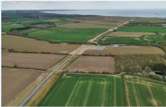
Part of the cable route from landfall at Ulrome.
