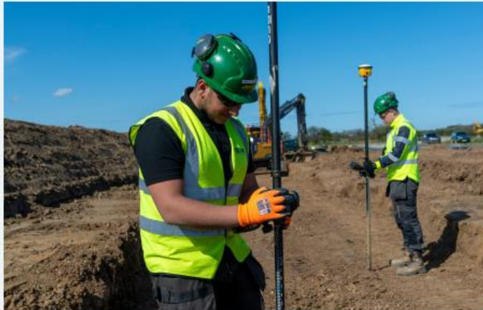
Engineers check the progress of the cable installation.
