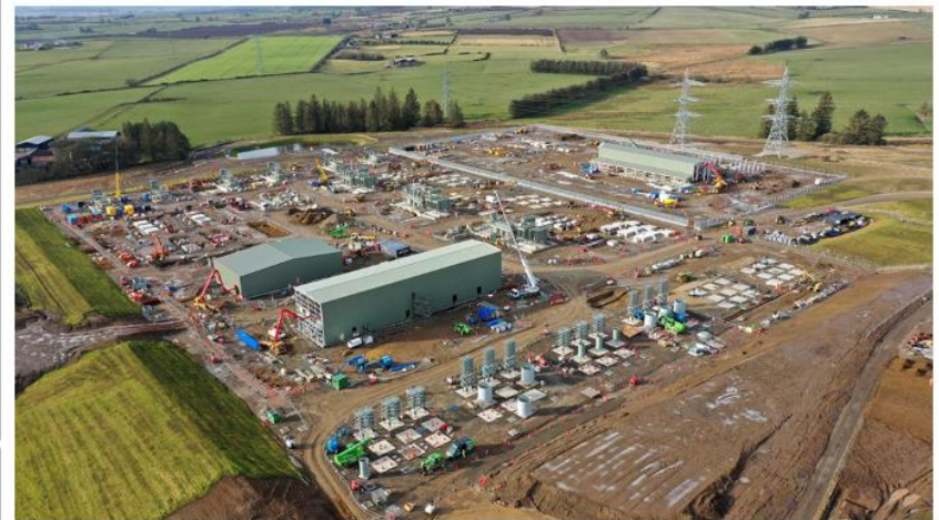
Substation site in February 2020
