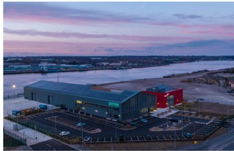
The Operations and Maintenance Base is now complete.
