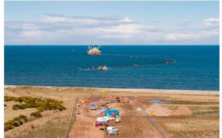
The cable installation vessel just offshore installing the export cables.
